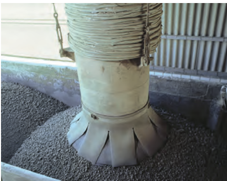
Bulk loading systems
