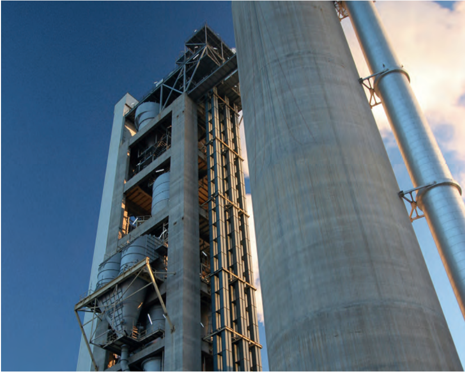
BEUMER bucket elevators are suitable for the vertical mechanical transportation of bulk materials, for example, in a cement works.
