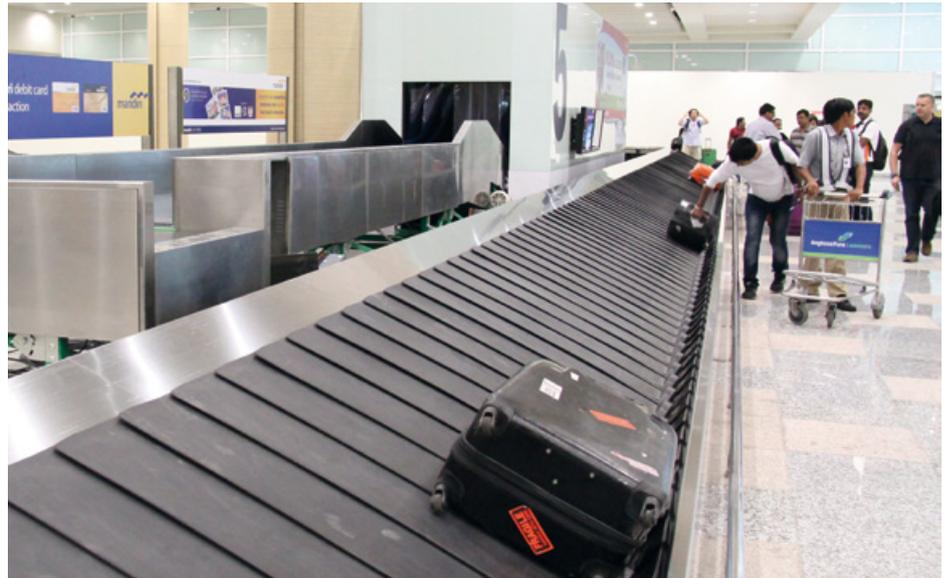
Depending on the total length, a carousel has one or more drive units. Carousel using two or more drive units can continue service with reduced load carrying capacity if one drive section fails. This redundancy comes from the principle of a self-adjusting friction drive. Integrated redundant drives automatically share the load if one drive section fails and baggage handling operations will continue uninterrupted.
