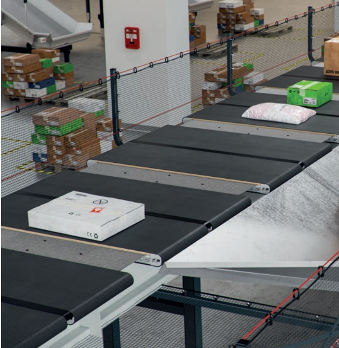
Smooth discharge into the package chutes
