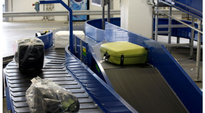
Loading in a conventional 'push' baggage handling system
