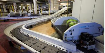
In a cart system, each cart carries a single piece of luggage. The system consists of a cart with wheels with a container-like carrier on top. The cart travels on a track like a roller coaster with a speed of up to 10 m/s and stops to load and unload.
