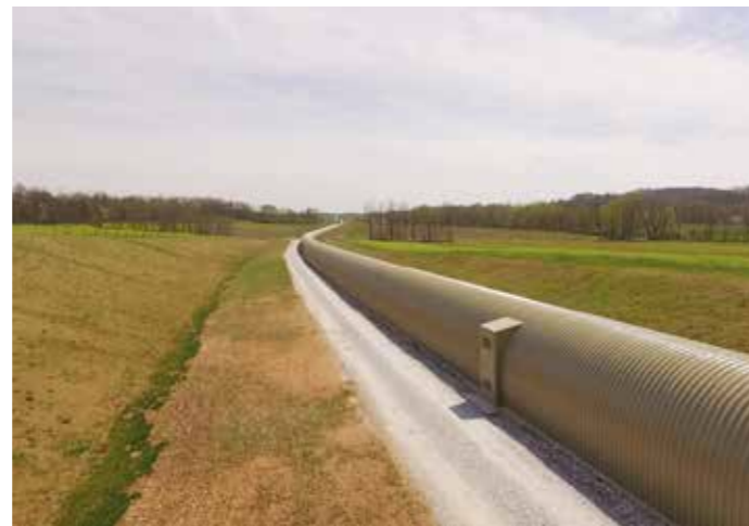
Horizontal Curve Trough Conveyor inside “Jumbo Covers”. The covers eliminate any exposure to the environment and provide ability to maintain the system out of the elements. There is room for a maintenance buggy to drive alongside the conveyor inside the covers.
