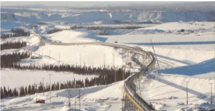
Overland conveyor for iron ore in permafrost, Canada
