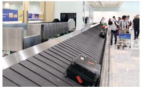
Depending on the total length, a carousel has one or more drive units. Carousel using two or more drive units can continue service with reduced load carrying capacity if one drive section fails. This redundancy comes comes from the principle of a self-adjusting friction drive. Integrated redundant drives automatically share the load if one drive section fails and baggage handling operations will continue uninterrupted.
